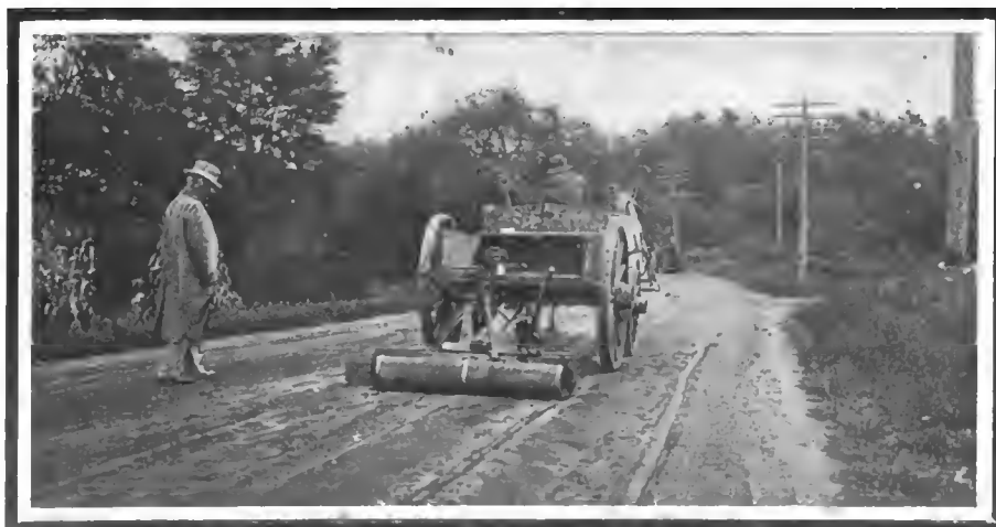
The small road roller and drag that are used in preparing roadbeds for their top dressing
